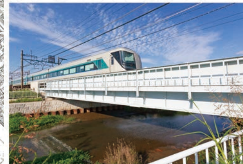
③ 姫宮落川橋梁
